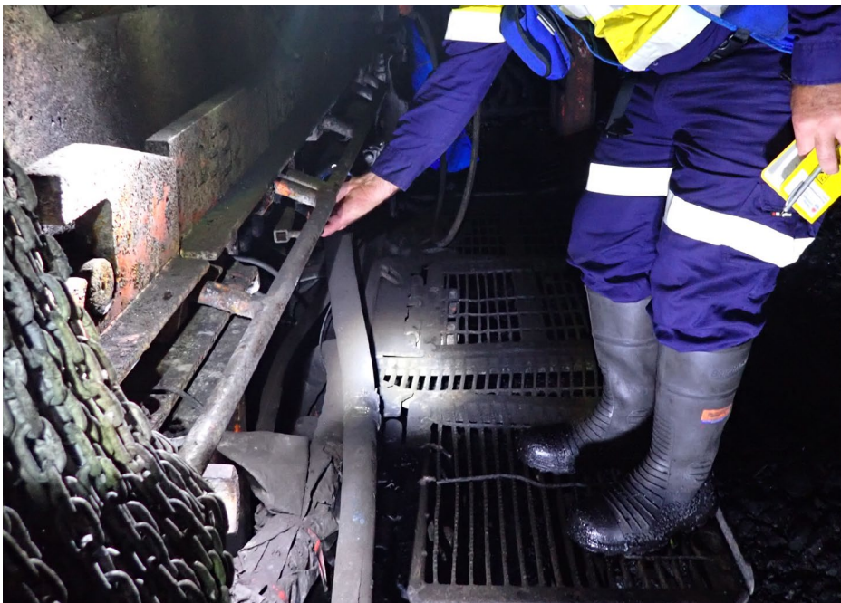
Figure 5 - Location of diversion valve above right side platform on CM313
