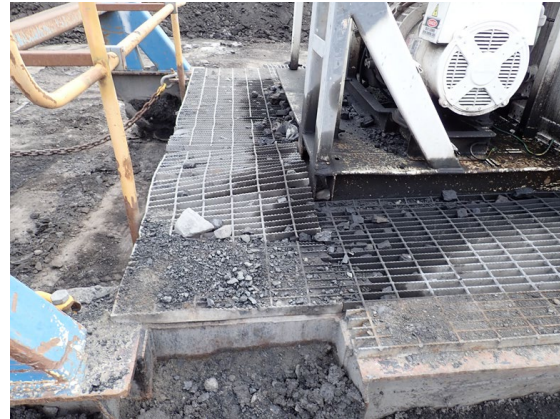
Figure 2 – Damaged platforms
