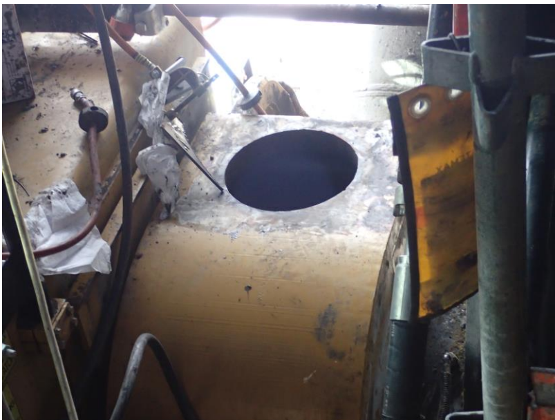
Figure 2: Superstructure void and test piece adjacent to access hole.
