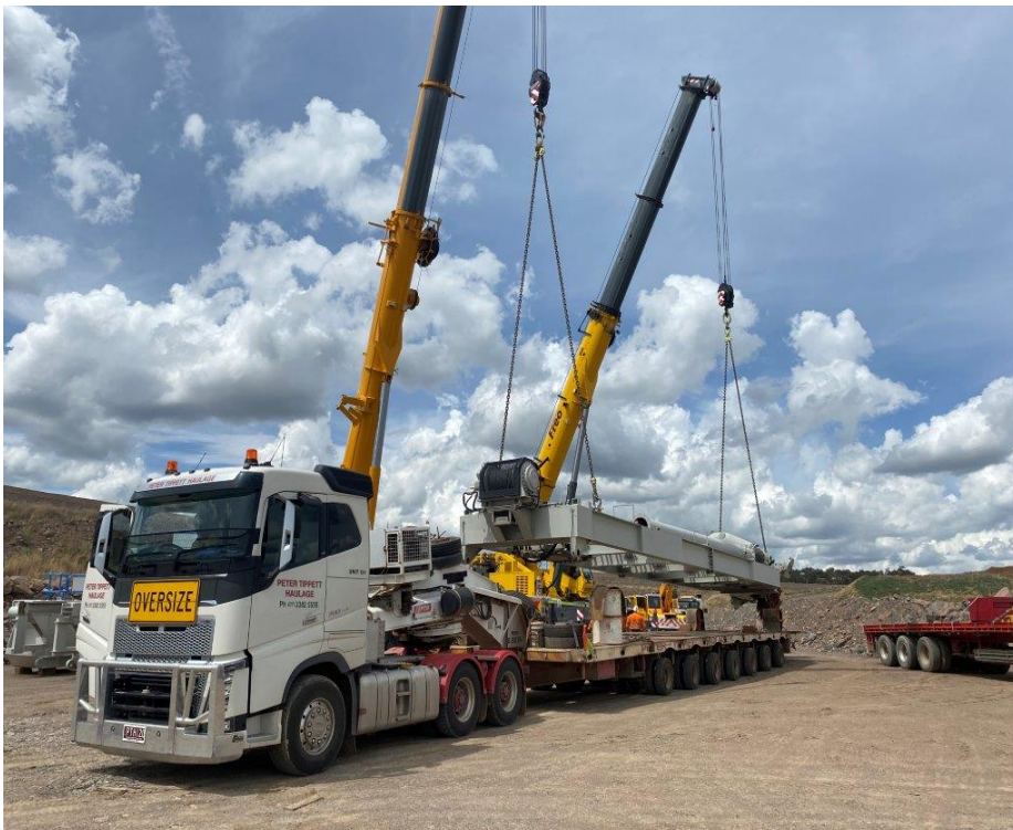
Figure 2 - Truck moved on placement of load
