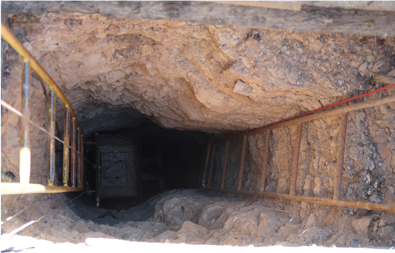
Figure 6: The steel bucket inside the hoist shaft
