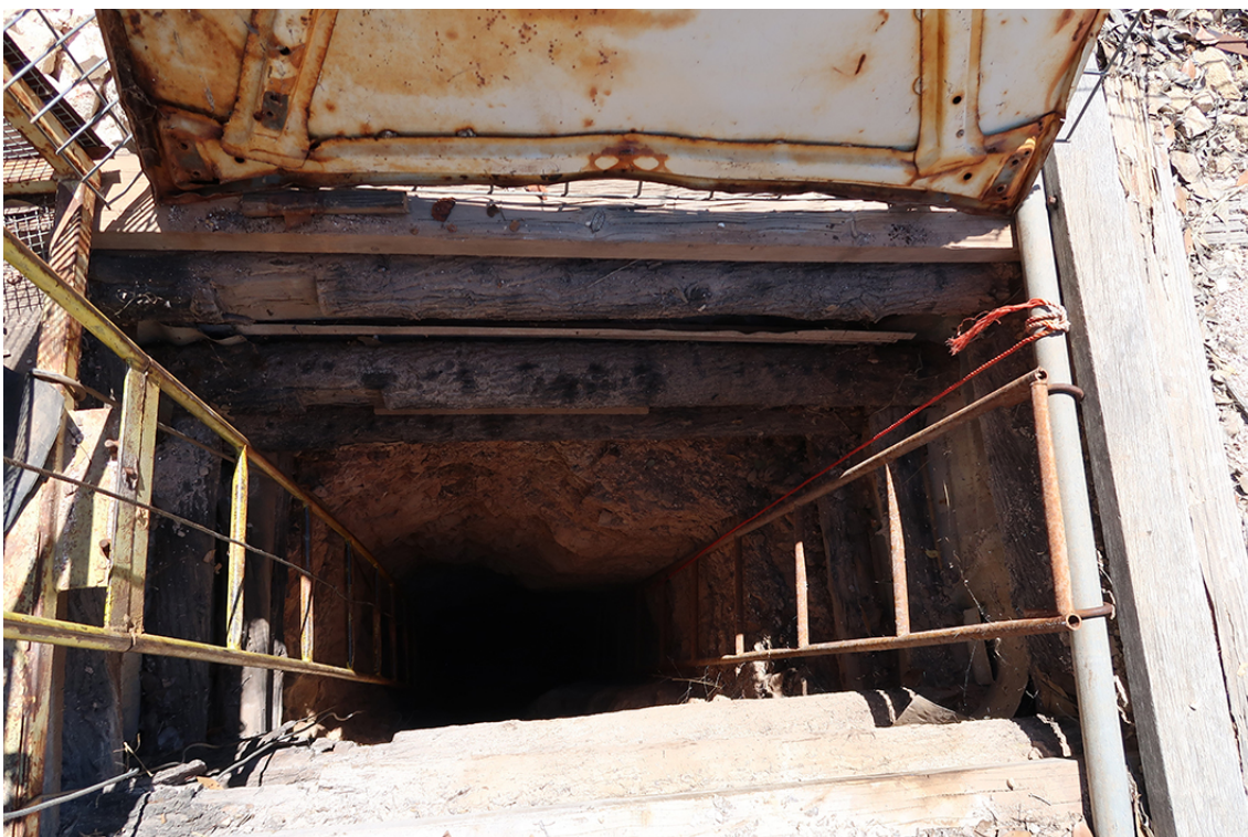
Figure 5: The entrance to the hoist shaft
