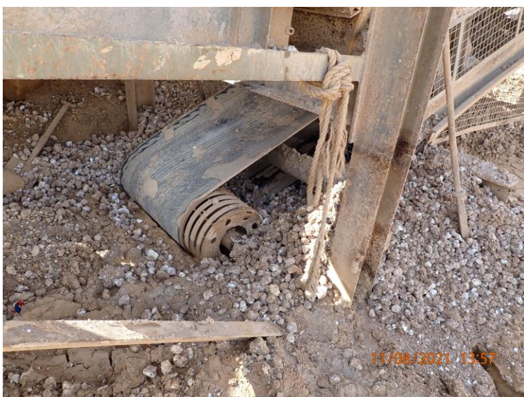
Figure 4: Unguarded tail pulley which was partially buried in loose material
