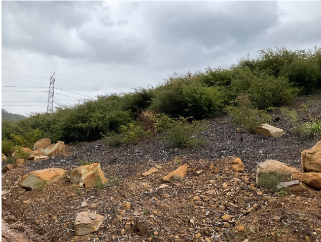
Figure 3. Part of the stockpile has been revegetated
