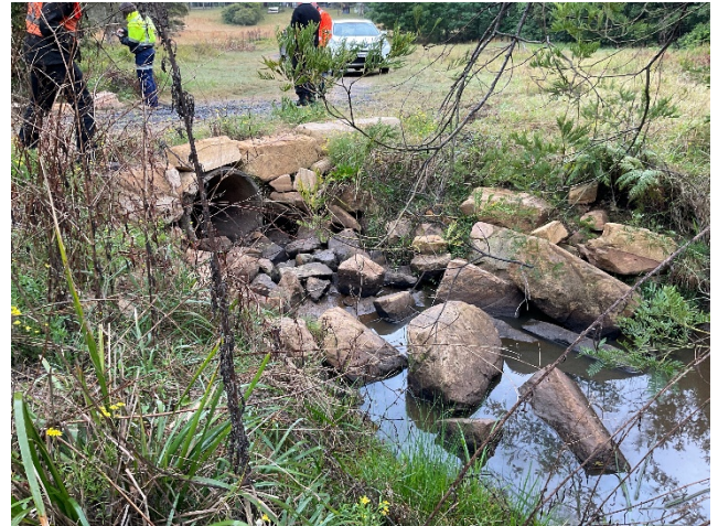
Figure 7. Drainage works to rectify subsidence impacts over LW26 in ML1722
