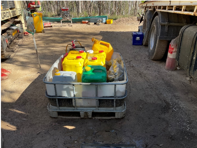
Figure 1. Secondary containment for chemicals, fuels and oils at site ELG157.
