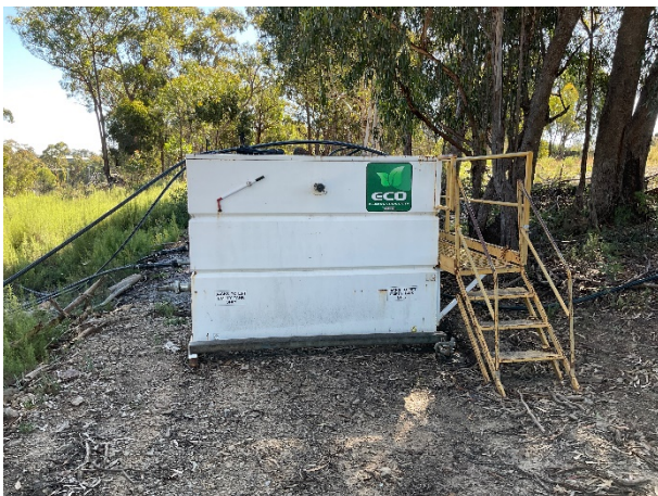
Figure 3. Aboveground sump being used to recirculate water for drilling.
