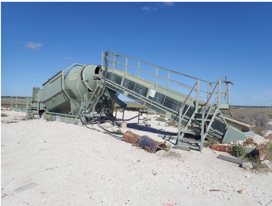
Figure 2: Agitator machinery with conveyor guarding, stairs and walkway
