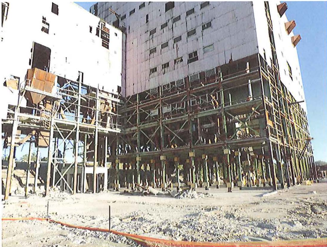
The Mill building ready for demolition
