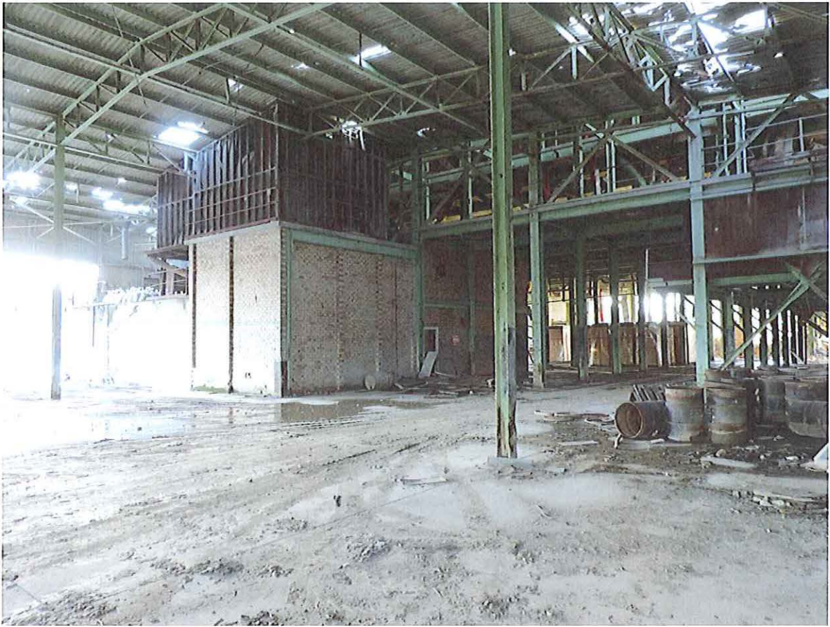
Brick section of the northern end of the mill building proposed for demolition 7 th Jan 2015
