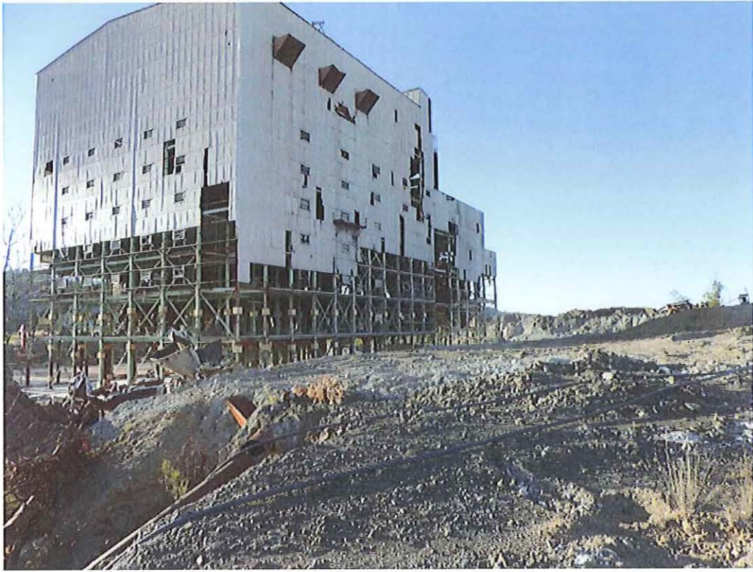
The Mill building ready for demolition
