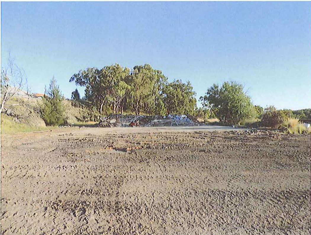
The Administration building demolished after the last inspection
